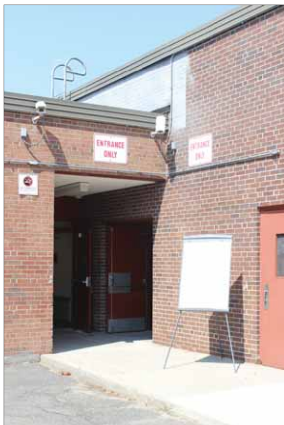
TURLEY PUBLICATIONS PHOTO BY GREGORY A. SCIBELLI There is a new main entrance to the high school located on the side of the building nearest the student parking lot.
